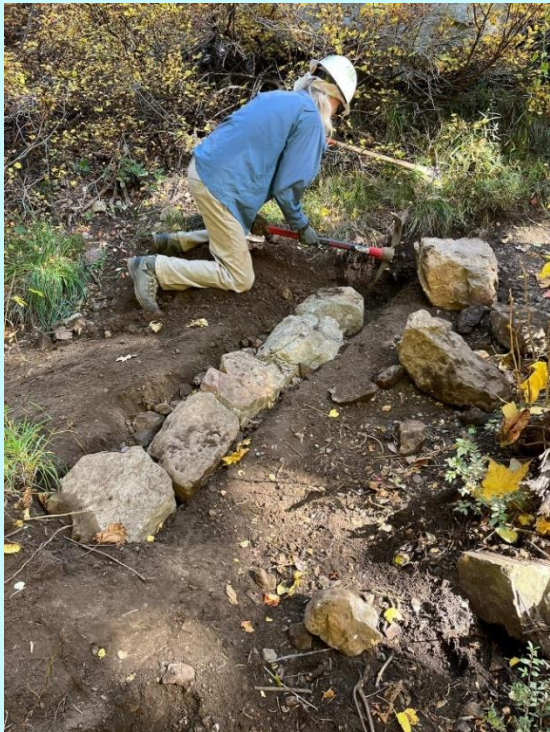
Photos of crew member Mike Roberts rebuilding water-bar style drains. Photo credits: Isaac Hodson
