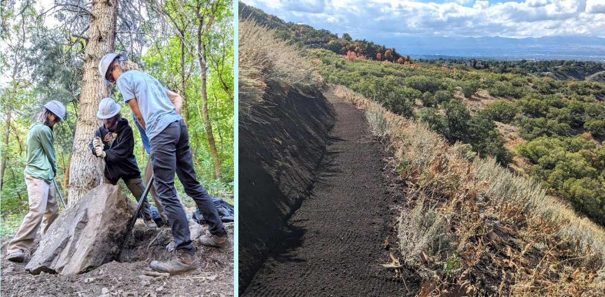
Left: crew members removing a rock from the tread. Right: newly widened tread above the valley. Photo credits: Emily Salle
