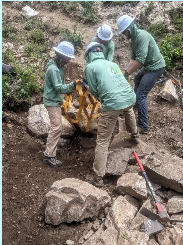
Above: the CCF crew moving one of the stair rocks into place. Photo credit: Emily Salle
