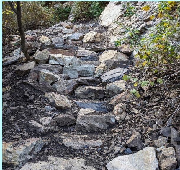
Some of the rock staircases installed along the approach and at the crag of Challenge Buttress. Photo credit Emily Salle.
