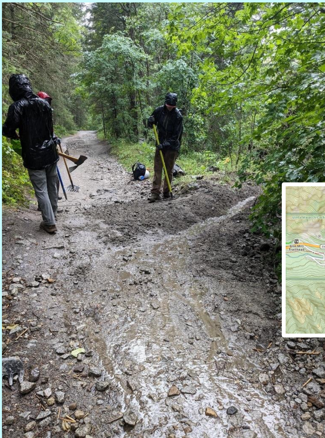
A rebuilt drain. Photo: Emily Salle
