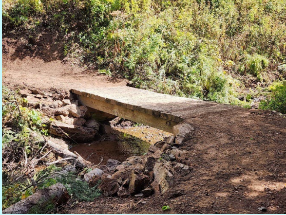
Bridge maintenance on the Great Western Trail. Photo credit: David Wyllie
