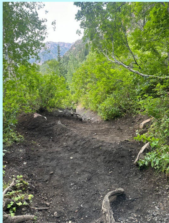
A rebuilt drain on the Lake Blanche Trail. Photo credit: Ryan Nordgran
