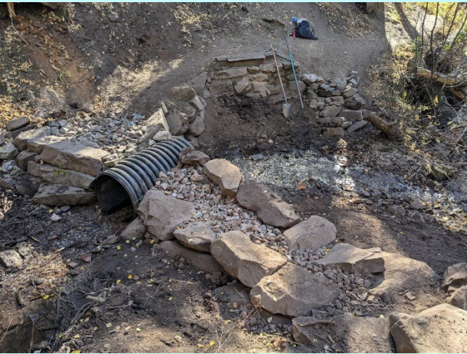
A series of photos showing the project development from the installation of the 18in culvert, to the triple layering of stone retaining walls, to filling the tread with crush and sediment. Photo credits: Emily Salle and Grace Goodwin-Boyd.
