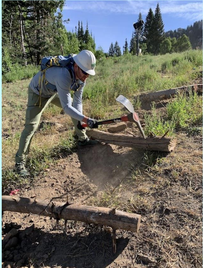
The old section of trail was restored with restoration checks, native plants, and debris. Photo credits: Grace Goodwin-Boyd
