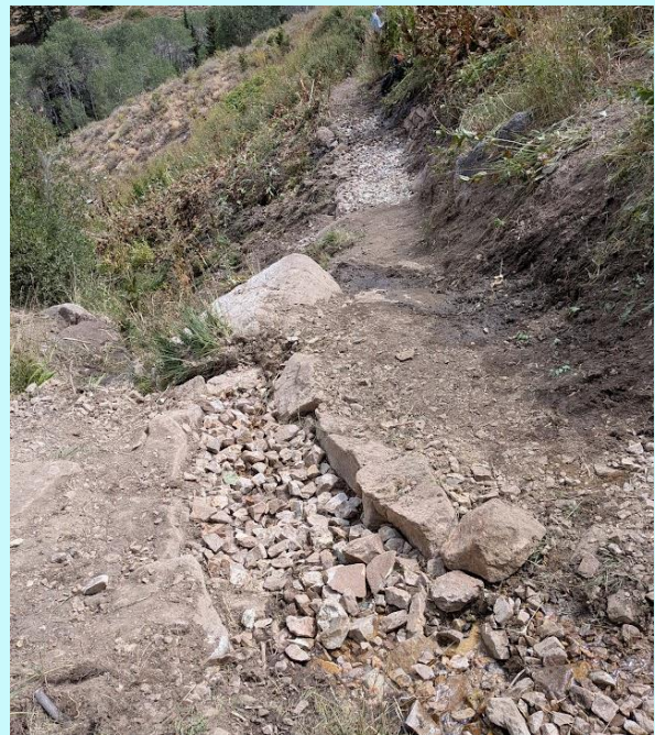
French drain, left, and open culvert on the Dry Lake-Pockets Fork Trail. Photo credit: Grace Goodwin-Boyd
