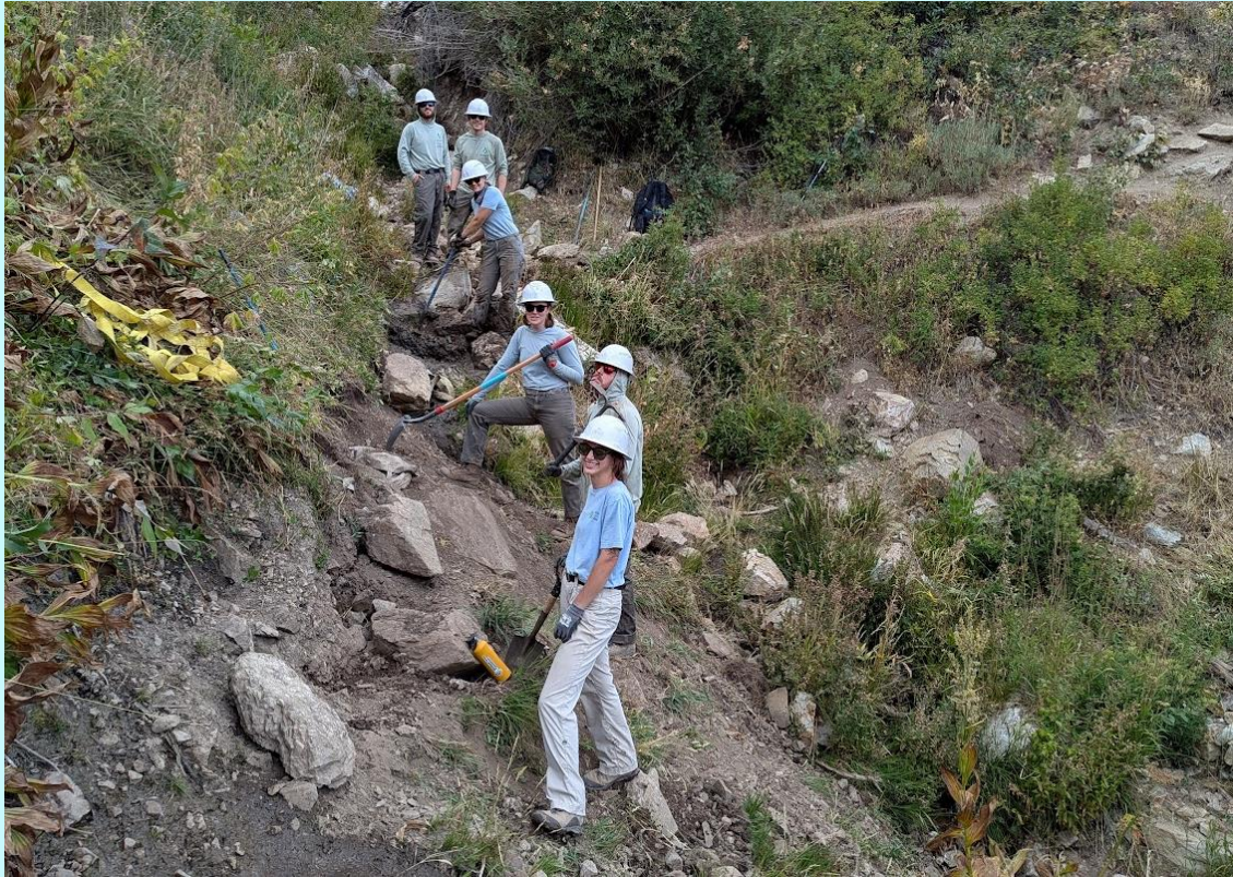
The CCF Trail Crew building drainage structures on the Deseret Peak Trail. Photo credit: Emily Salle.
