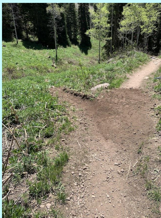
A cleared drain on the Lake Desolation Trail. Photo credit: Grace Goodwin-Boyd
