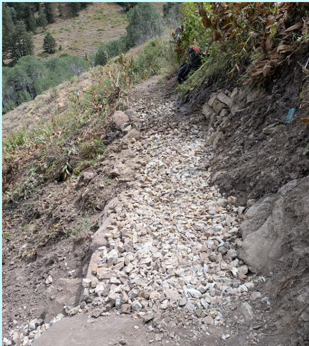
French drain, left, and open culvert on the Dry Lake-Pockets Fork Trail. Photo credit: Grace Goodwin-Boyd
